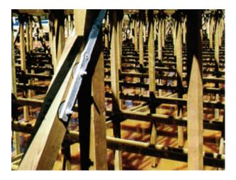
Transverse fan deck and hot water basin girts are 2" x 6"—all other transverse girts and all longitudinal girts are 2" x 4" except where loading may require 3" x 4". Transverse and longitudinal girts are spaced on 6'-0" vertical centers. Girt lines are through bolted to the columns.
