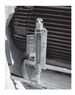
Fans of the size used on large cooling towers are applied at speeds and horsepowers that generate considerable torque — and structural tubular steel resists this torque most effectively. The Marley torque-tube assures that all of the
