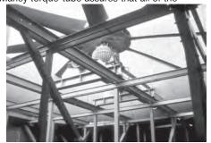
Open, gravity-flow distribution basins are a feature of crossflow type towers that adds to their reputation of being simple to operate and easy to maintain. These basins are out where they can be easily inspected even maintained—while the tower is in operation. Spray systems of counterflow towers, sandwiched between the top of the fill and the drift eliminators, are comparatively awkward to access, and require tower shutdown for maintenance.
