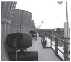
fan cylinder segment shall be through-bolted to both the fan deck and a primary fan deck framing member. Anchorage by lag screws into the fan deck alone will not be permitted. Fan cylinder connection and anchorage hardware shall be series 300 stainless steel.
